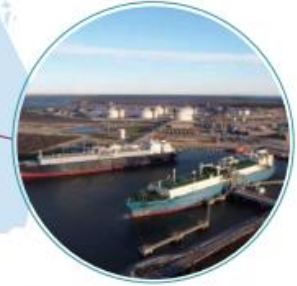
Sabine Pass Liquefaction ~30 mtpa Total Production Capacity
